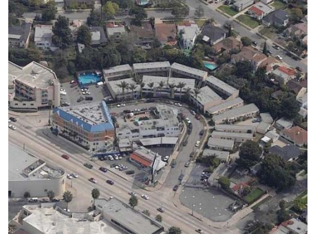
Existing 1 and 2 story structures
