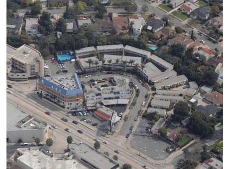
Existing 1 and 2 story structures
